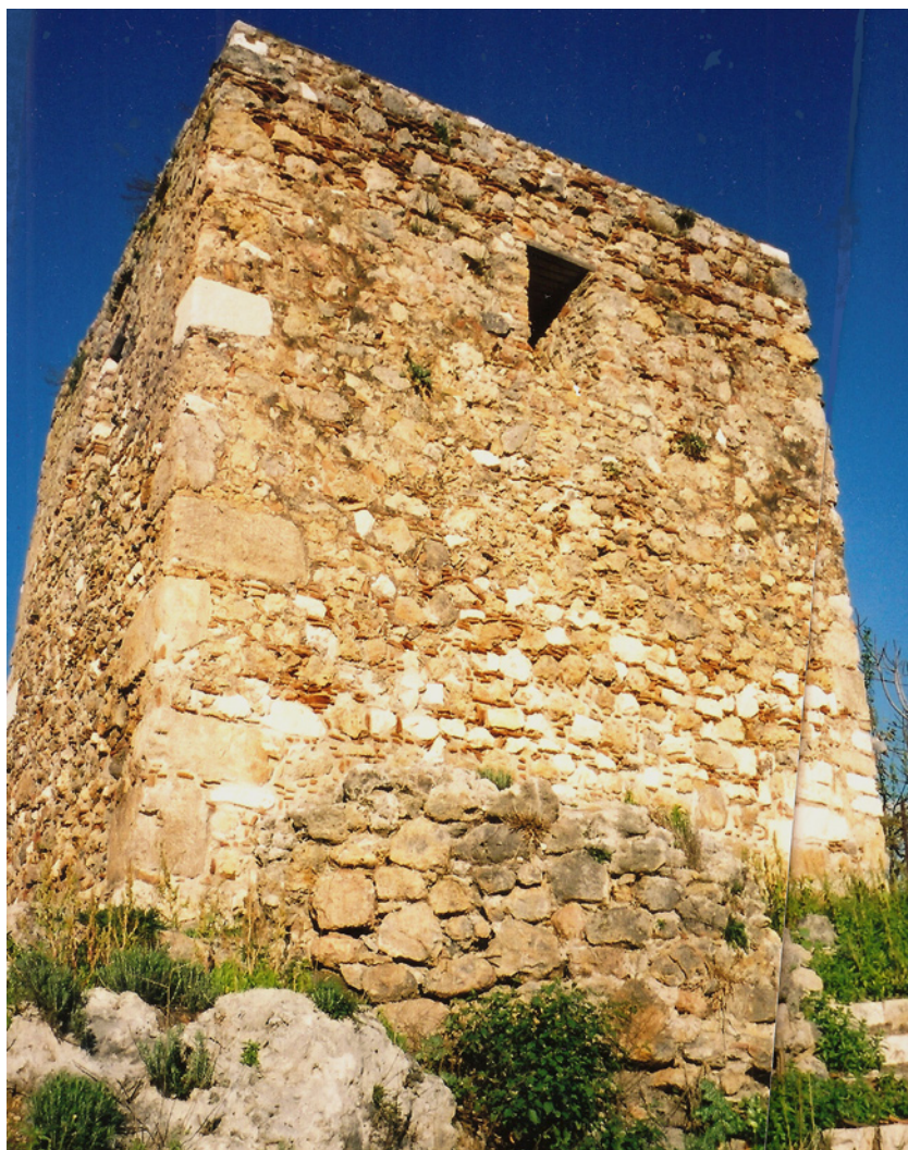
Fig. 221. Katochi. S façade of the tower.
